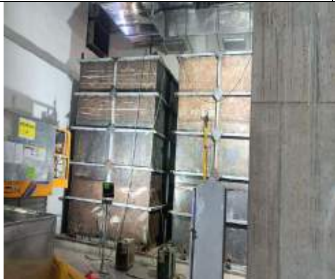
STP Under Construction
