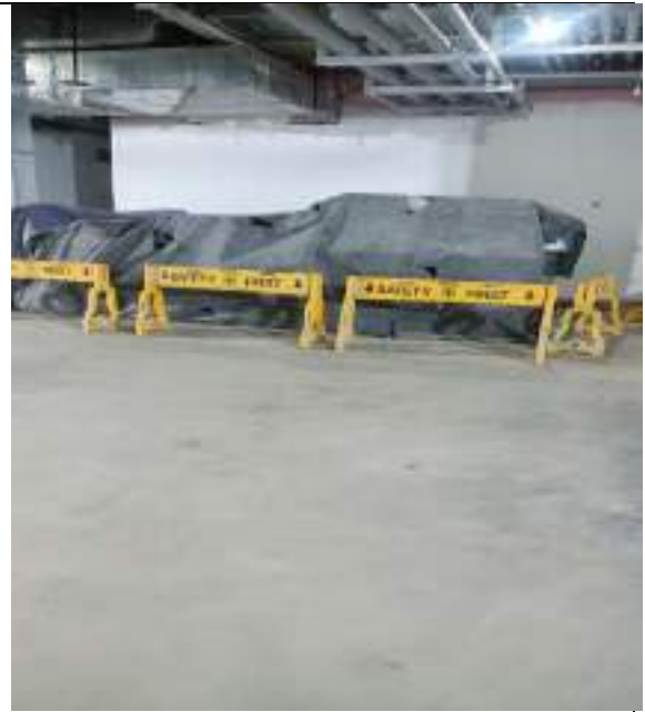
Barricading With Covered Material at site
