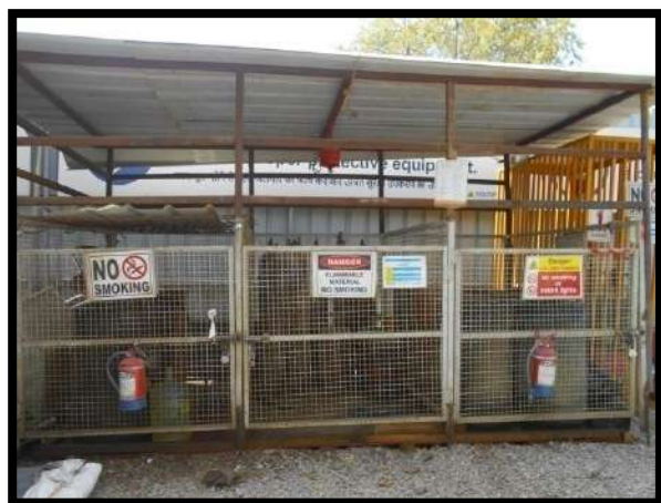
Figure 2.12 Isolated Diesel Storage Area
