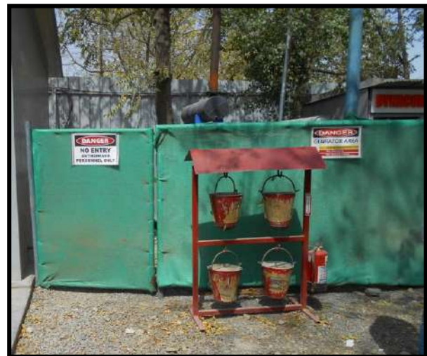
Figure 2.2. Fire Fighting Facility
