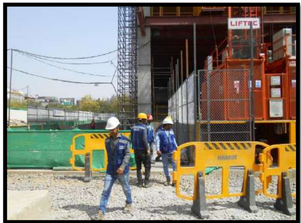
Figure 2.10 Workers with PPE
