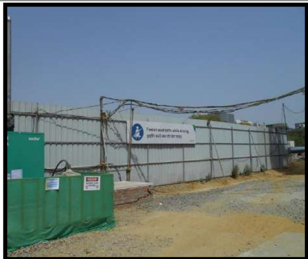
Figure 2.6. Barricading at the Project site
