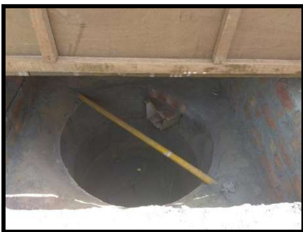
Figure 2.11 Provision of Storm Water Control
