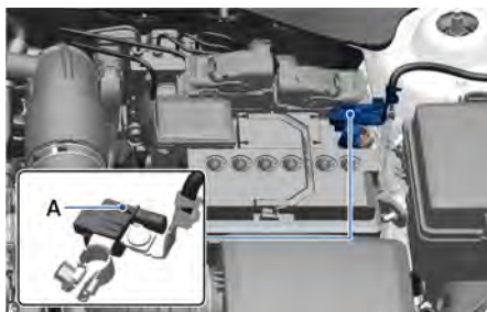
[A] Battery sensor
