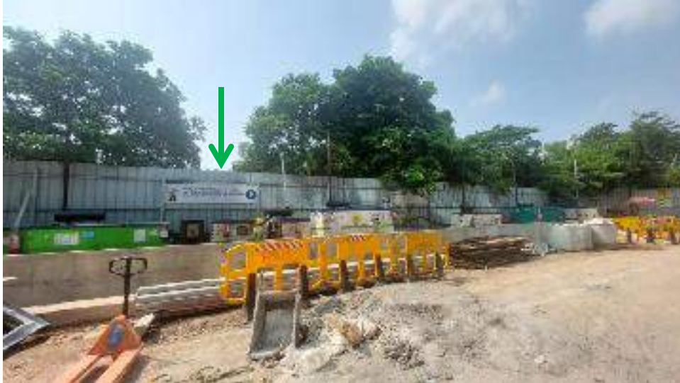
Barricading Around the Construction Site
