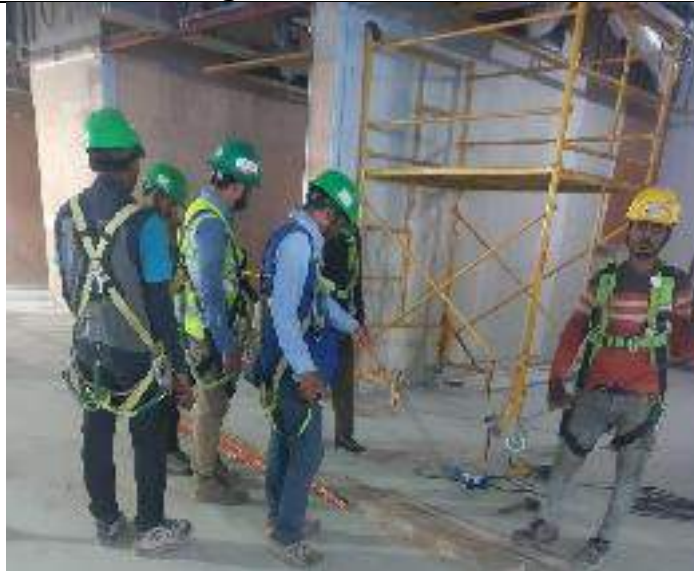
Workers Equipped with PPE
