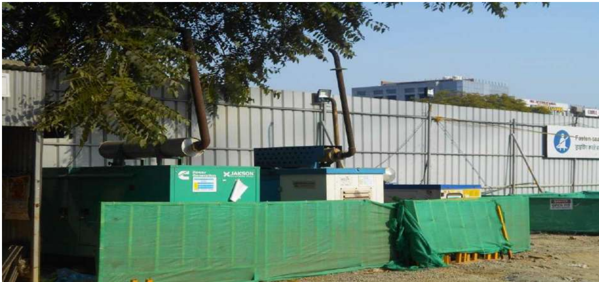
Figure3.5 DG Set photograph
