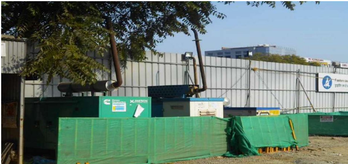
Figure3.5 DG Set photograph
