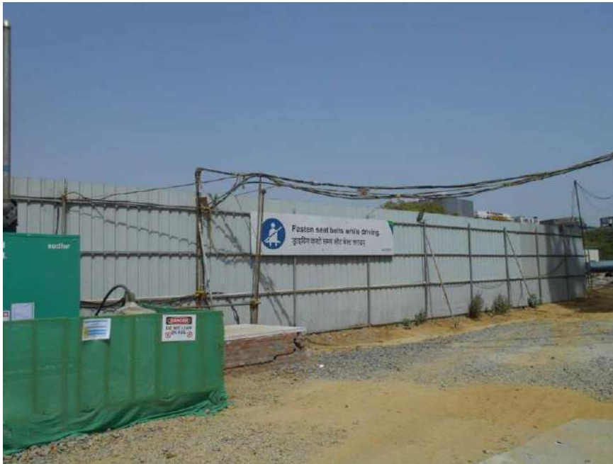
Figure3.2 Barricading all along the boundary of the project site
