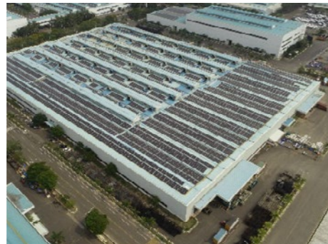
A photovoltaic power generation facility in HMI
