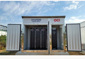
300kWh commercial ESS at the OCI Plant
