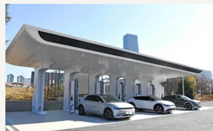
E-pit charging station
