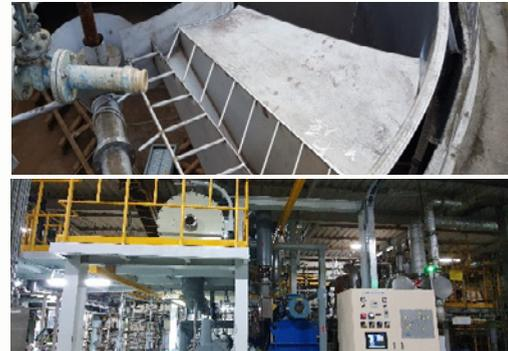
Above. Dissolved Air Flotation installed at the paint shop 52 of the Ulsan Plant
