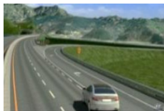
Highway TG Entry/Exit
